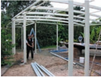
The Pavilion next to the building takes shape.
